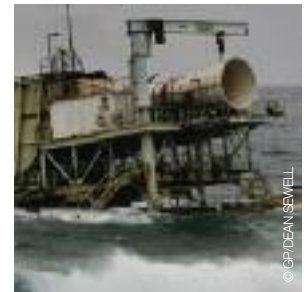
image Wave power technology using a column of water to drive a turbine.
